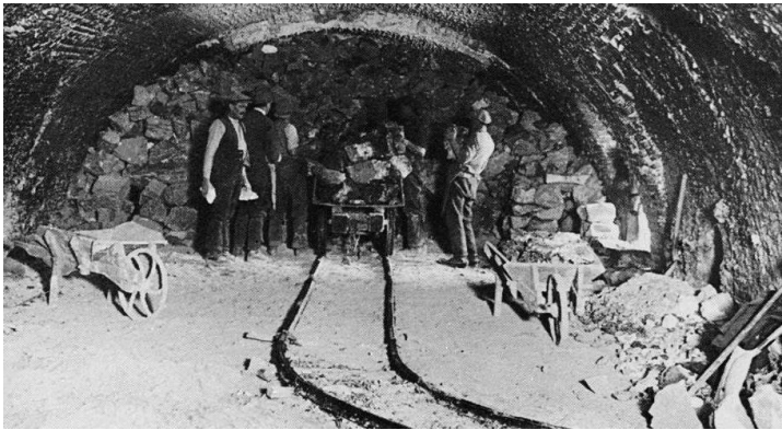
Fig 17: Stone loading into the Hoffmann kiln at Harpur Hill, Buxton
