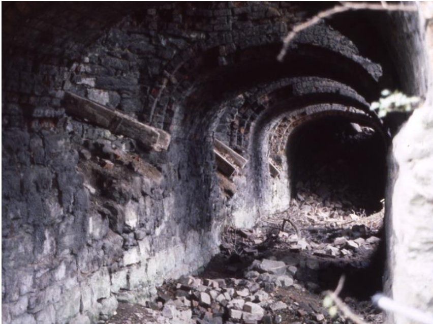
Fig 10: Remains of the wooden chutes used to transfer quicklime directly from the Bellman kilns to railway trucks
