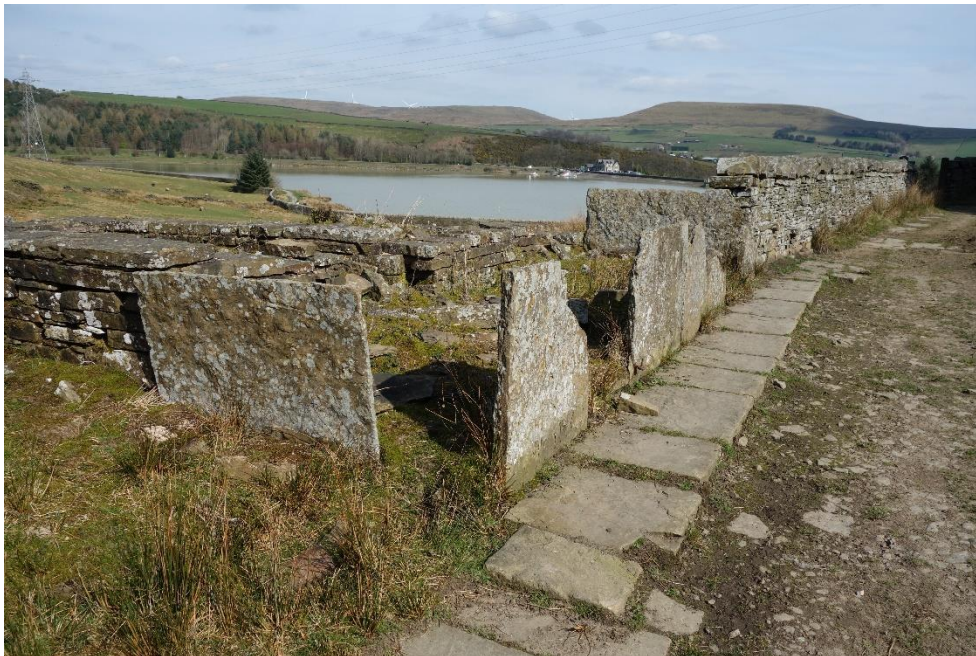
Thin sandstone slabs used as fences. Cown Reservoir as backdrop.
